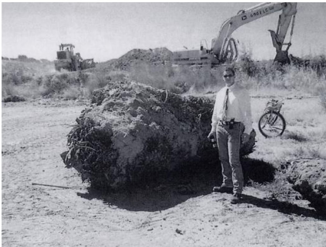
Figure 2. Buried mass excavated in dredge ponds at Mare Island. Contents of such masses include welding rods, silverware, china, tools, and a wide range of UXO.
